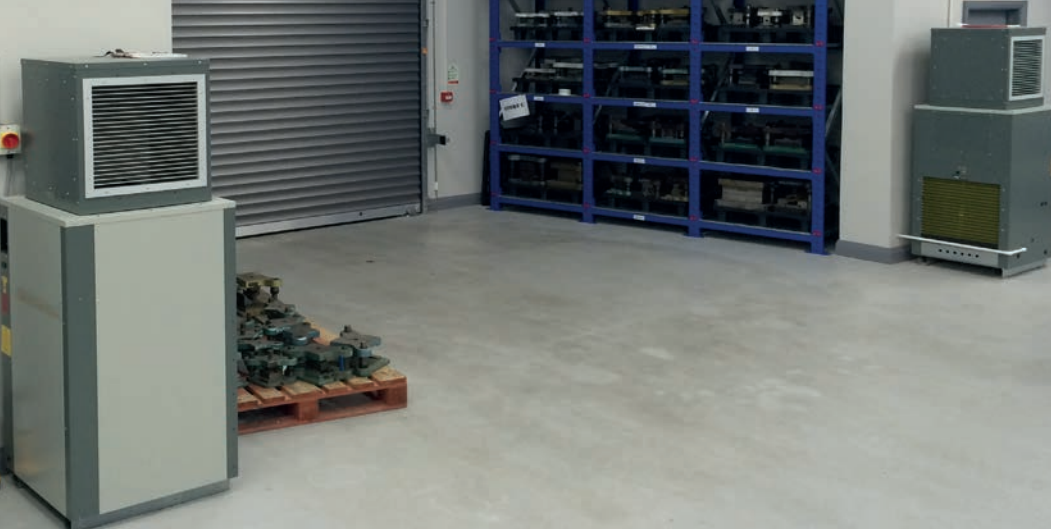
Two Calorex DH150 dehumidifiers maintain the humidity within the Preci-Spark storage facility
